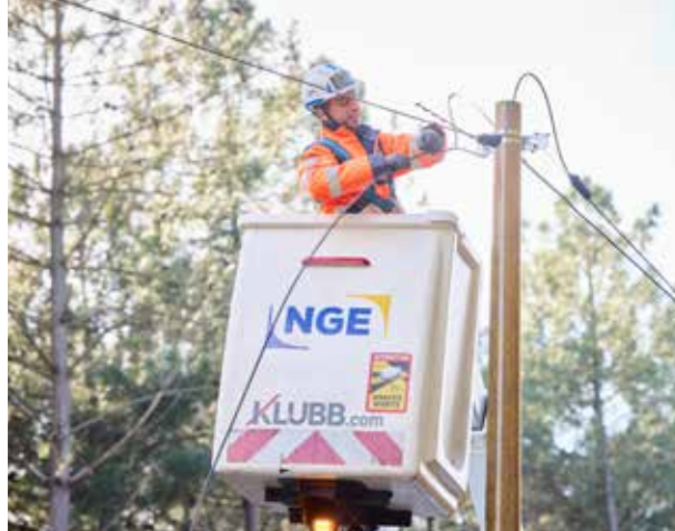
▼ Installation of fibre in Gironde
