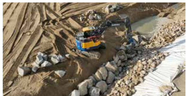
▼ Reinforcement of the sea defence structure in Jullouville
