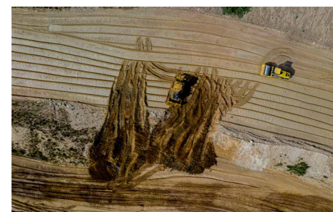
Bypass of Baraqueville by the RN88
