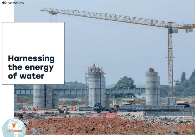
Temporary sluiceways allow water from the Sanaga River to flow  $\P$  through the site during construction of the Nachtigal hydropower plant in Cameroon
