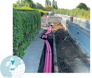
The first trenches are dug for the Liverpool optical fibre ▶ rollout
