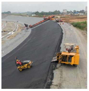
The 35-metre beam paver applies waterproof surfacing **T** to the Nachtigal Dam power channel
