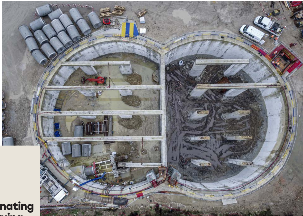
Rainwater treatment plant in Champigny sur Marne
