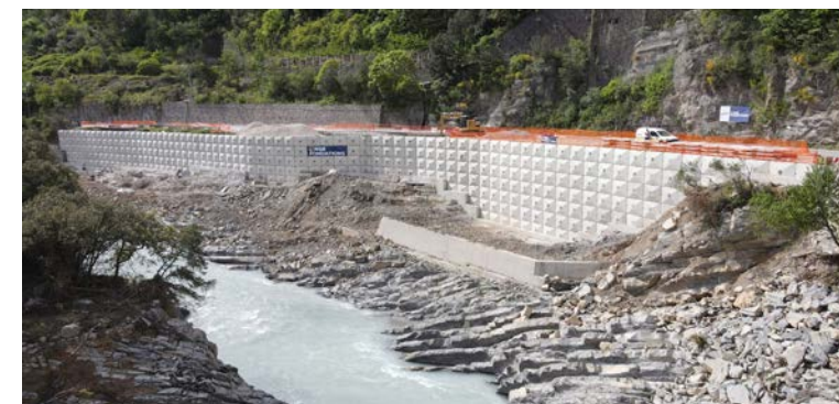
AD/OC® nailed wall, Roya Valley
