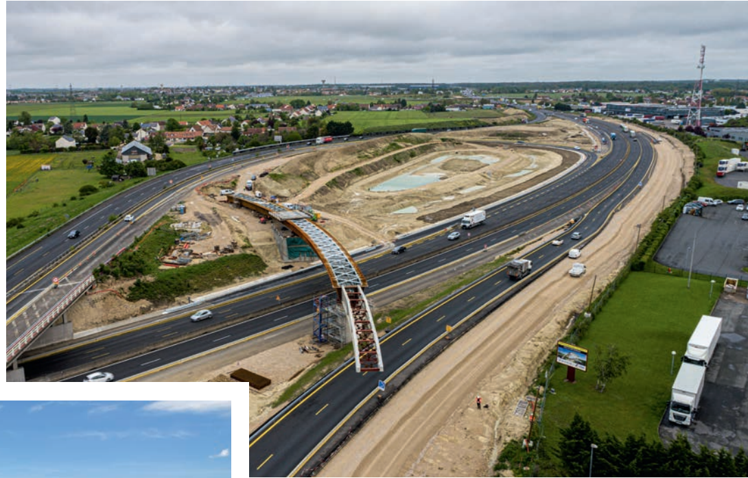
▲ Development work underway on the A10/A71 junction.
