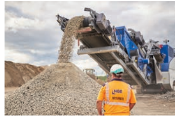
▲ The waste recovery platform in Martignas-sur-Jalle was one of the first in the Group. This image shows concrete crushing operations.
