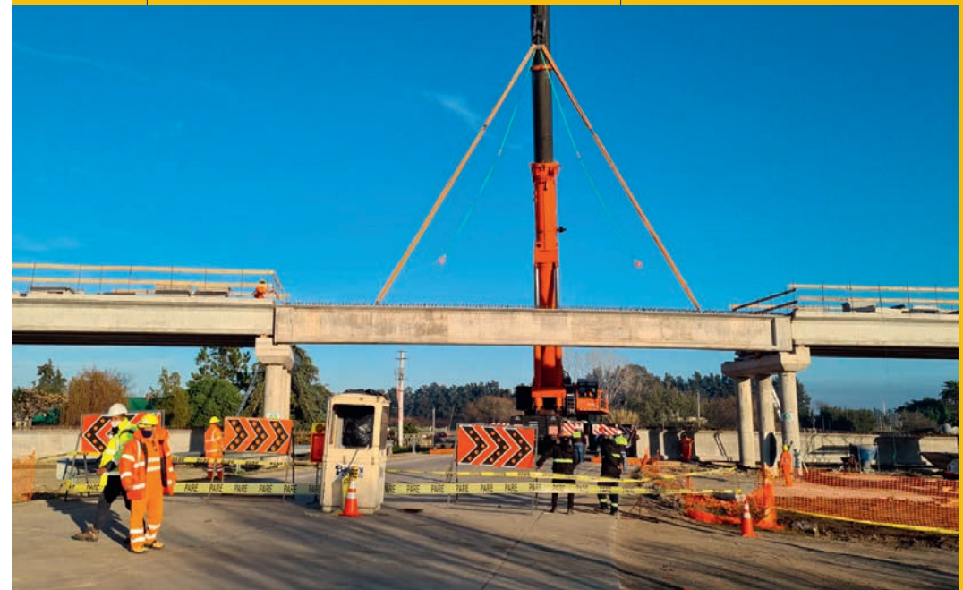
▲ Installing a beam for a rail bridge in Uruguay.
