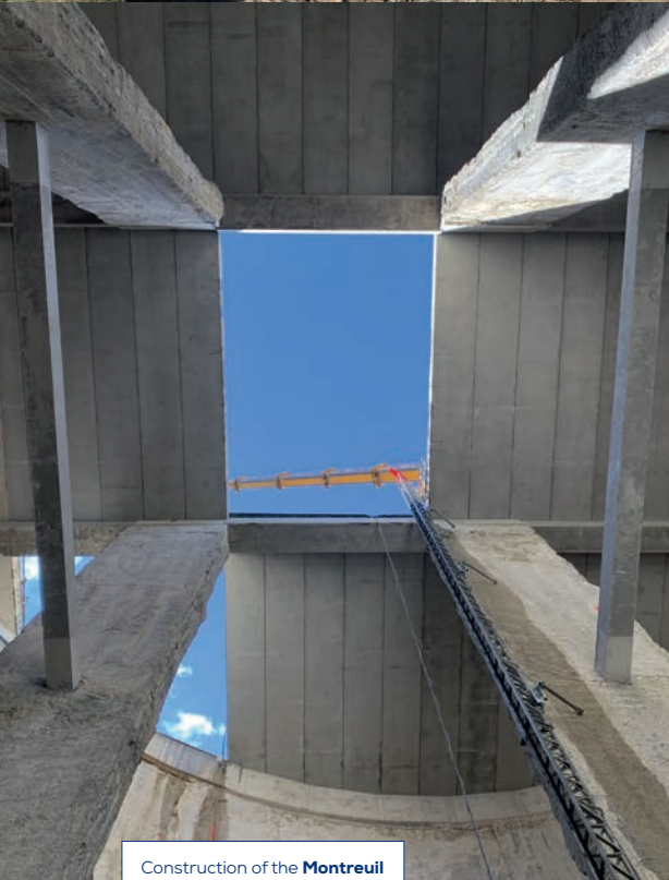
Construction of the Montreuil stormwater holding tank
