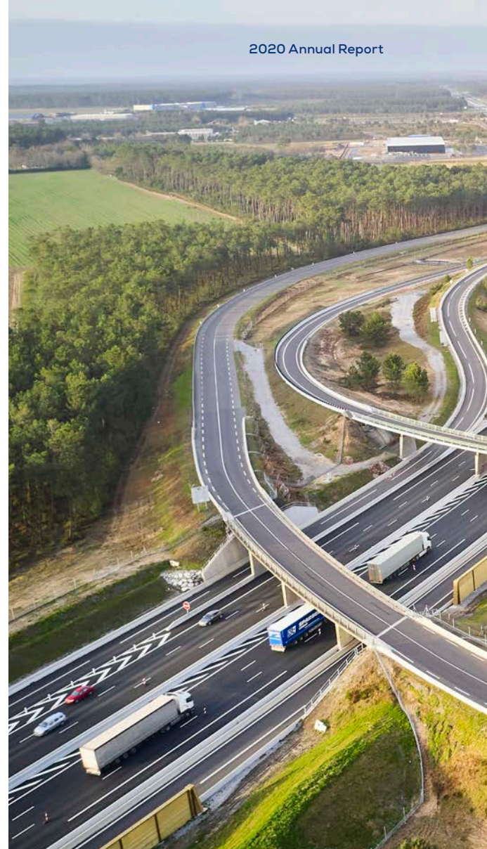
▲ The A63 between Bénése-Maremne and Saint-Geours-de-Maremne in the Landes department.
