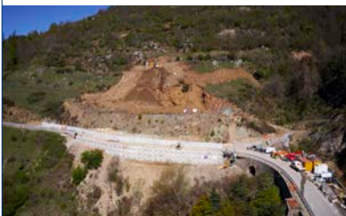
▲ The traditional solution of shotcrete was replaced by prefabricated concrete slabs to create 306m 2 of AD/OC® walling.
