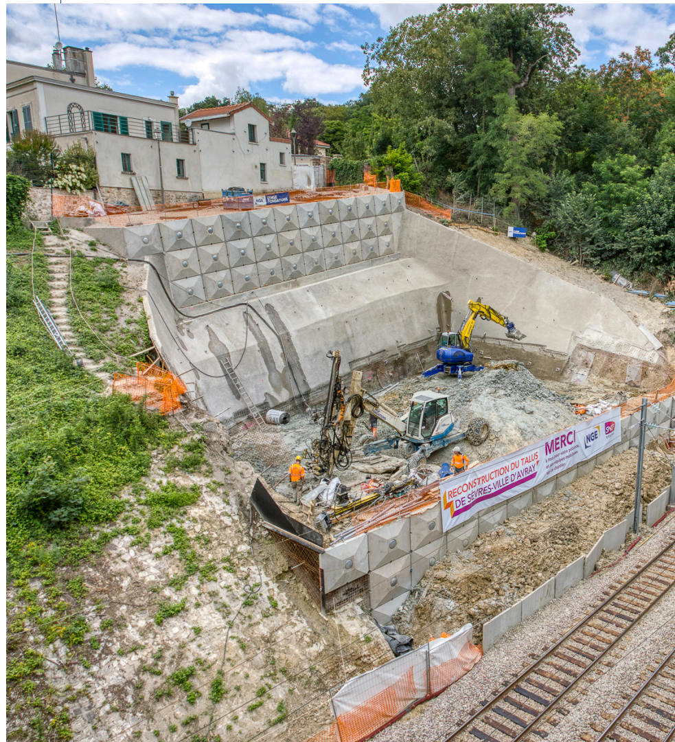
▲ The traditional solution of shotcrete was replaced by prefabricated concrete slabs to create 306m 2 of AD/OC® walling.
