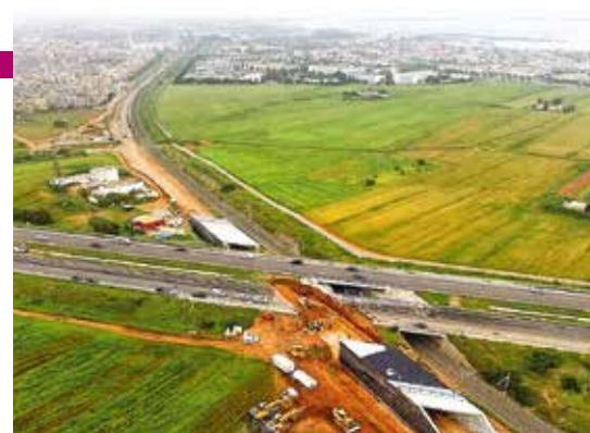
/ Slide-in bridge construction on the work site to triple the rail track between Casablanca and Rabat in Morocco
