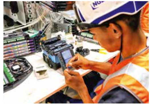
/ Optical fiber installation and connection
