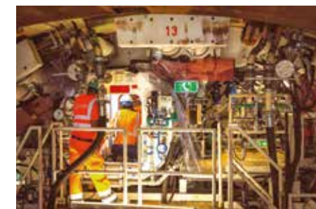
/ The Grand Paris project - Tunneling machine at work on Line 15
