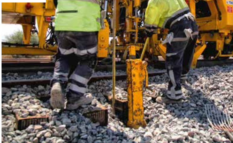
/ Rail ballast undercutting in Mexico
