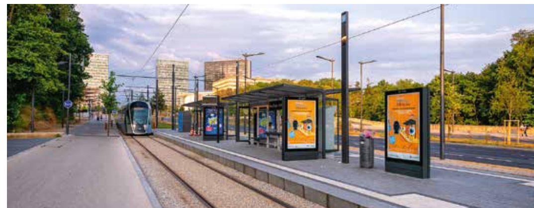
/ Construction of the Caen tramway
